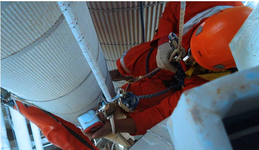
Fig. 1. PEC CUI examination of a vertical pipe using rope access operator to cut down scaffolding costs and reduce preparation time to access the object
